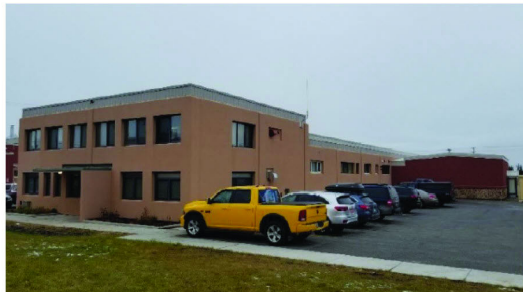
e. Fort Greely Bldg. 603, Directorate of Public Works Headquarters (northeast corner)
