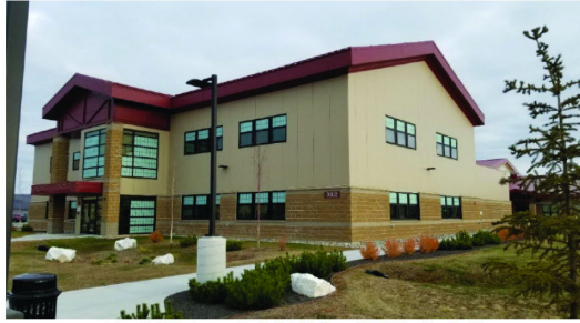
a. Fort Wainwright Bldg. 3002, Aviation Battalion Headquarters
