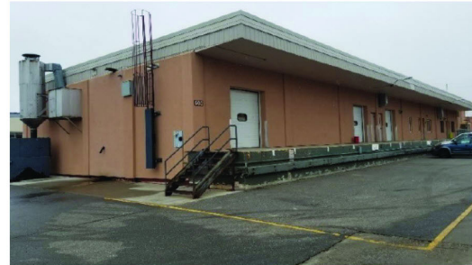
d. Fort Greely Bldg. 603, Directorate of Public Works Headquarters (southwest corner)
