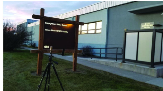
f. Fort Greely Bldg. 650, Theater and Gross Motor Facility
