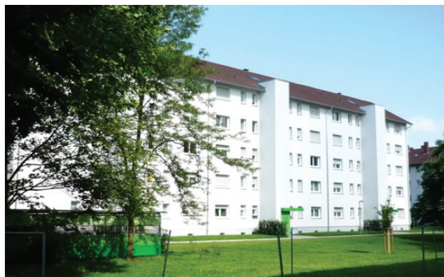
Figure 1 Exemplary refurbished multi-family block of flats from three analyzed buildings in Karlsruhe-Rintheim (Source: VOLKSWOHNUNG GmbH).
