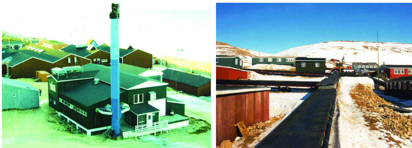
Figure 9 Heating system in Quaanaaq, Greenland: (a) combined heat and power (CHP) plant (cooling fans are used only for emergencies), and (b) above-ground utilidors.
