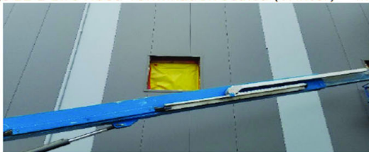
Image 11-4 IMP Louver Termination Sealed
