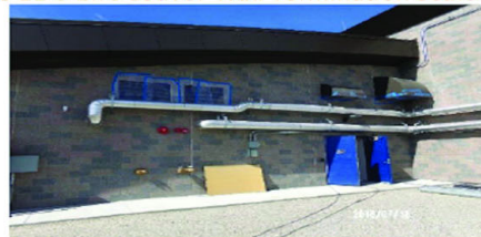
Image 11-5 CMU Louver Wall Termination Sealed
