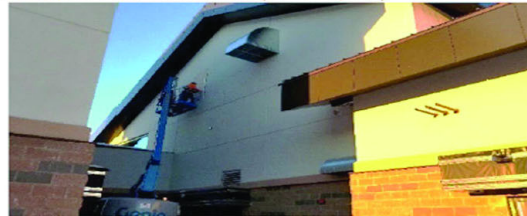
Image 11-3 EIFS Louver Wall Termination Sealed (Winter)
