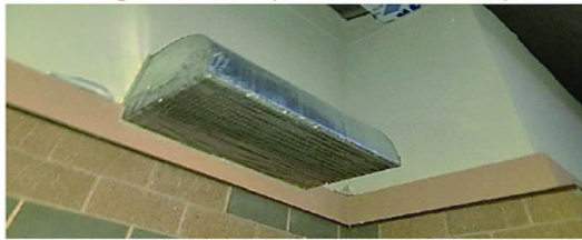
Image 11-2 EIFS Hood Termination Sealed (Winter)
