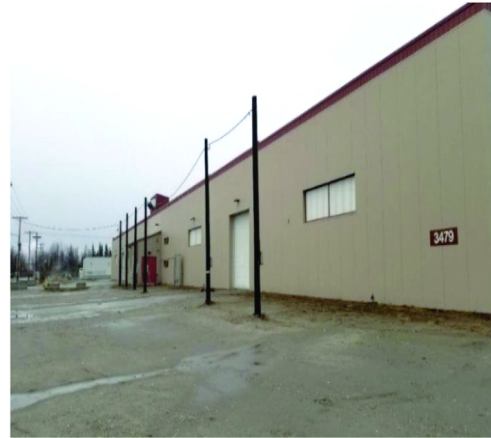
Image 9-2. Building 3 Storage Facility and Shop
