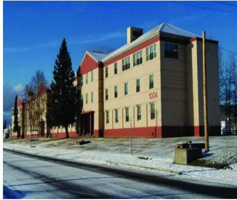
Image 8-1. Building 2 Concrete Wall/Steel Roof
