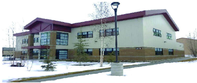
Image 2-1. Bldg. 24,26 Typ. Construction
