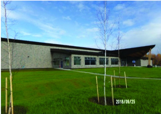
Image 5-1. Bldg. 27 CMU Wall & Metal Roof
