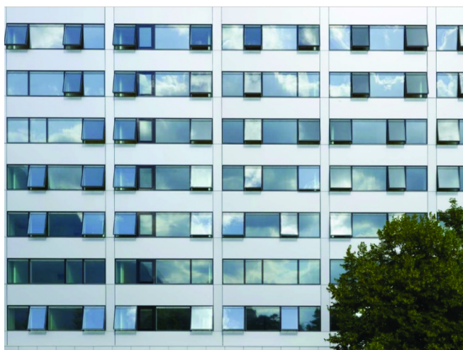
Figure 4 New façade with automated window opening for ventilation on the main building at Campus Technik. (Source: ATP architekten ingenieure, Innsbruck architekten.)
