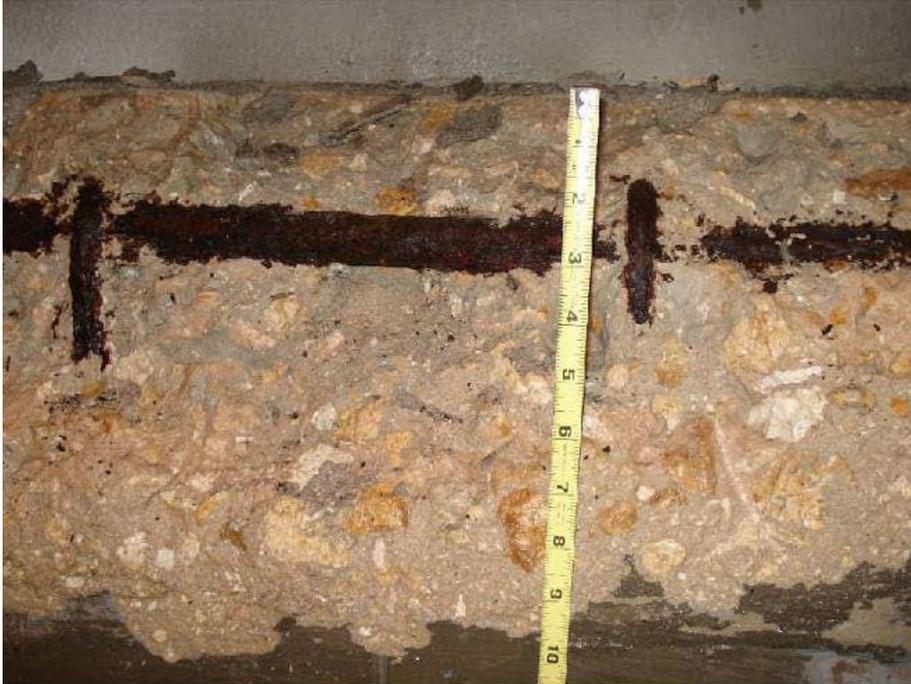
**Figure 4-15. Shows a typical section of exposed corroded rebar.**
