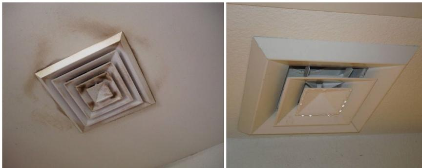
Figure 5-18. Condensation on ceilings and diffusers.
