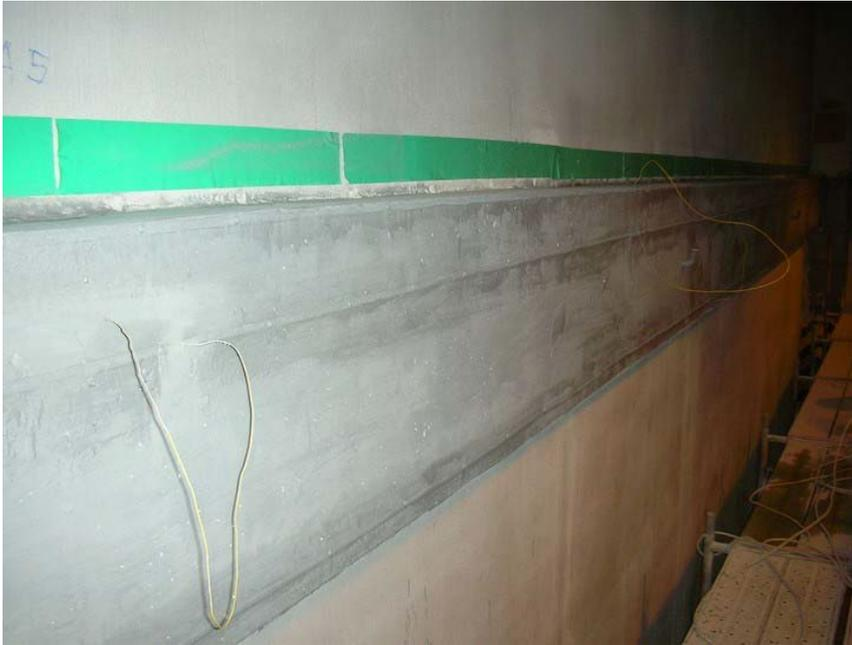
**Figure B-16. Finished appearance of the Ring Girder Side 2 following application of the LGC.**
