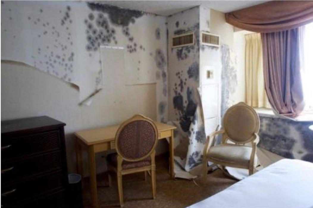
**Figure 4-5. Moisture trapped by an interior vinyl wallpaper vapor barrier.**
