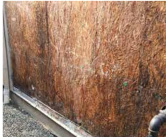
**Figure 1-5. Example of saturated-oriented strand board (OSB) sheathing.**
