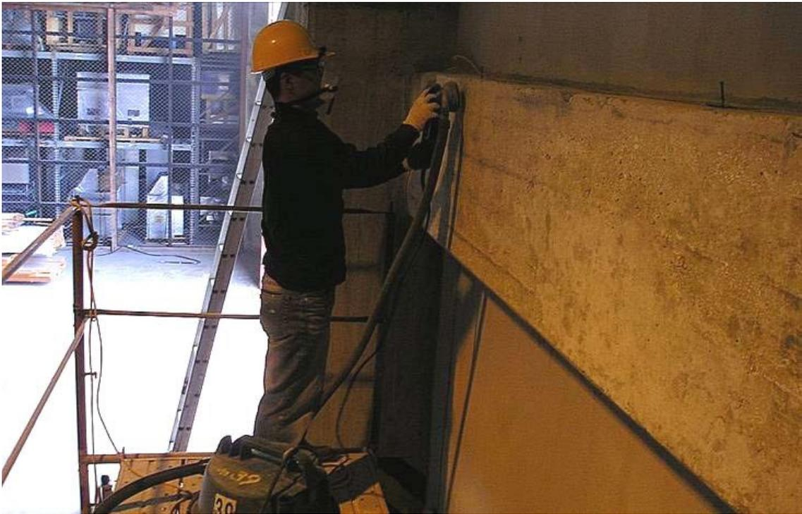
**Figure B-3. Failed existing repairs; new delaminated areas were demolished.**
