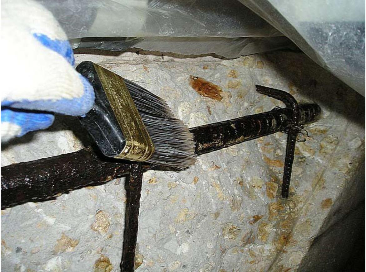
**Figure B-6. Organic vapor phase corrosion inhibitor applied to all demolished delamination areas.**
