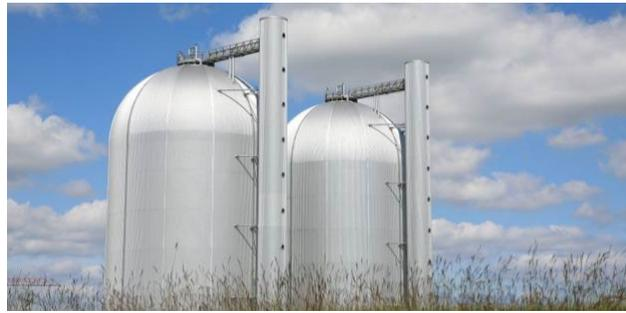
2 x 24,000 m<sup>3</sup> pressurized hot water TTES in Copenhagen Denmark, up to 257.0 °F (125 °C) sectioned from network by 10 Bar (Ramboll)
