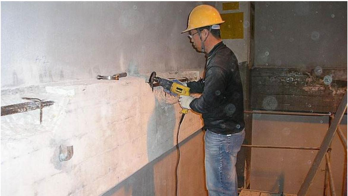
**Figure B-5. Exposed rebar in repair areas cleaned by using wire wheel.**
