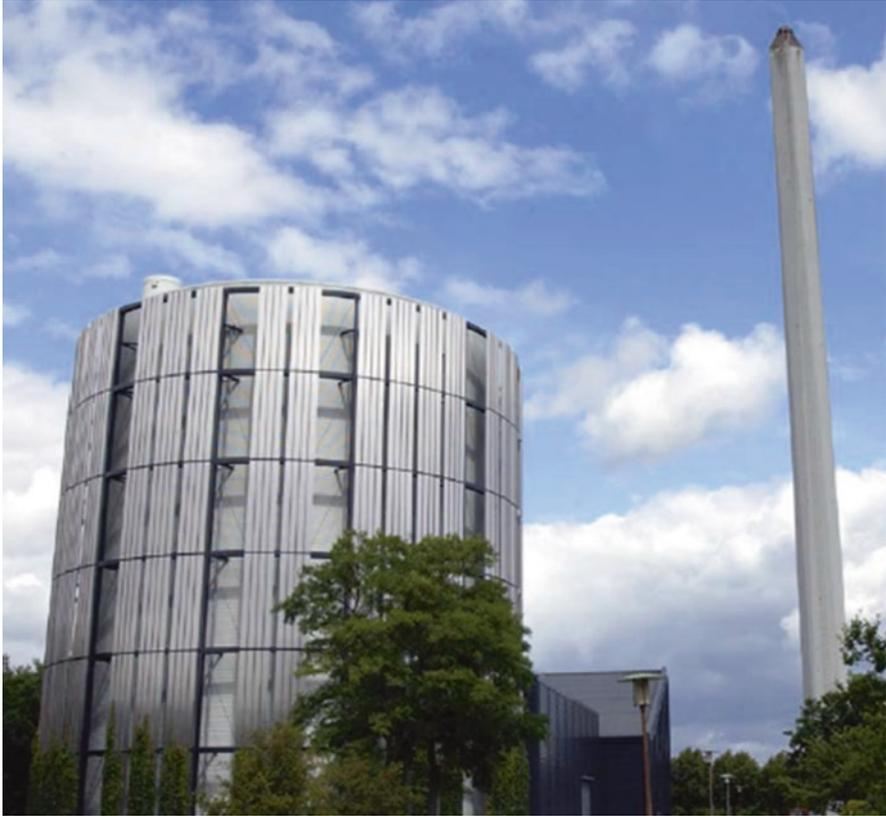
**Fig. 7.17** Hot-water storage tank with a capacity of 8000 m<sup>3</sup> (2823 ft<sup>3</sup>), ready to use
