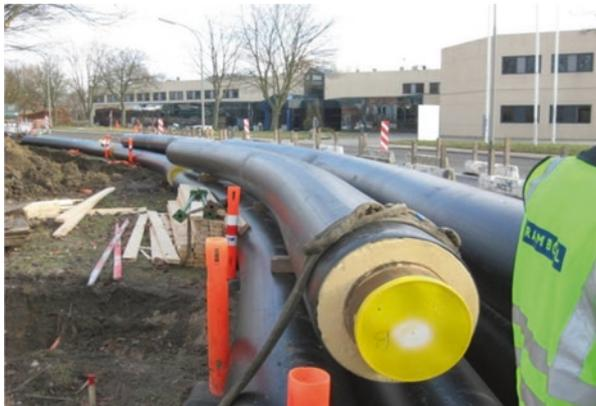
Fig. F.61 Installation of pre-insulated pipes
