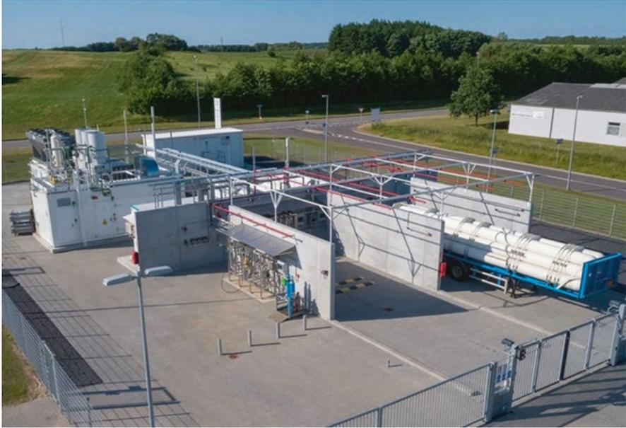
**Fig. F.87** Power-to-gas facility in Hobro. (Source: [https://www.dgc.dk/sites/default/files/filer/publikationer/C1703\\_IGRC2017\\_iskov.pdf](https://www.dgc.dk/sites/default/files/filer/publikationer/C1703_IGRC2017_iskov.pdf))
