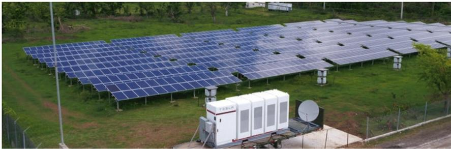
Fig. 7.10 Emergency power generation using a PV panel field connected to a battery pack
