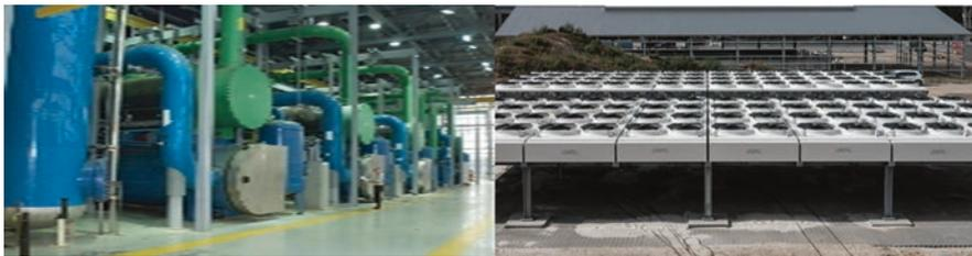
**Fig. F.50** Electric chiller and air coolers
