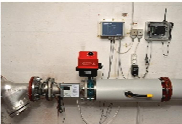
Fig. F.74 Dantaet pressure section (leakage protection)
