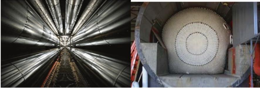
**Fig. F.90** (left) Utility tunnel for district heating pipes between Rigshospitalet and Amagerværket in Copenhagen, (right) tunnel plug developed by DHS S&T
