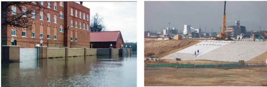
**Fig. F.89** Masonry floodwall in Fargo, MD (left); armored levee in Japan (right)
