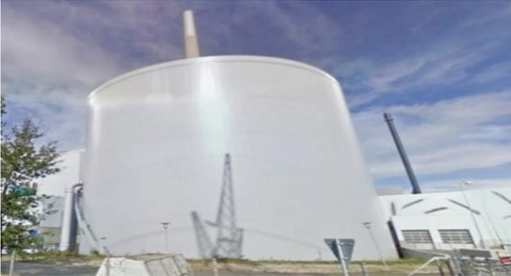
**Fig. F.52** The largest tank is probably the 75,000 m<sup>3</sup> (2,648,600 ft<sup>3</sup>) pressureless hot water storage tank in Odense Denmark owned by Fjernvarme Fyn
