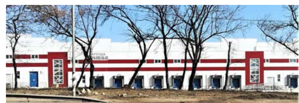
Figure 2. Multiple gates of a warehouse building.
